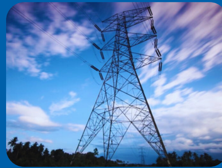
Transmission Tower Projects
